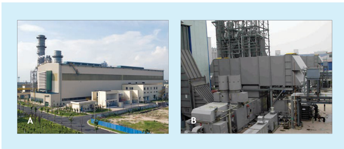
Figure 12: (A) Frame 9E.03 operating on steel mill gases at a plant in China; (B) LM2500+ operating on high H_2 coke oven gas.
