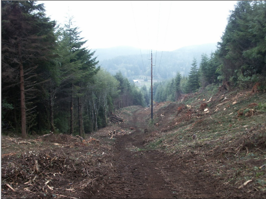
Figure 6.1. In densely vegetated areas, rights-of-way usually have to be completely cleared initially to establish a wire-border zone.
