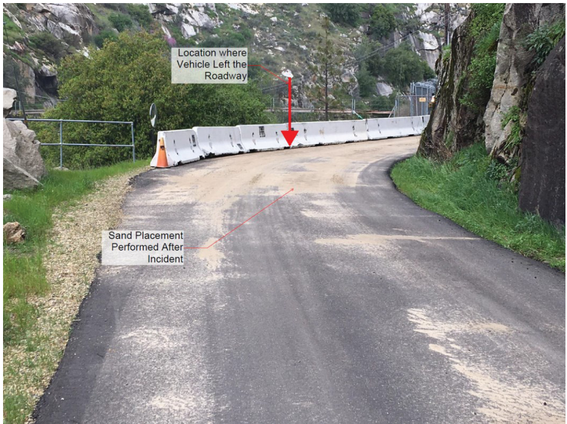
Figure 2 Post Incident: Temporary concrete barriers and traffic mirror installed along incident road curve location. Note: Direction of photo is facing east and the sand on the roadway was laid down after the incident.
