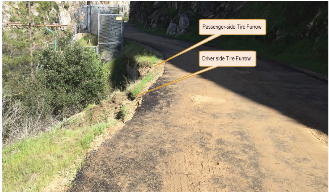
Figure 3 Vehicle exited road while traveling east (Note: Direction of photo is facing east and the sand on the roadway was laid down after the incident).
