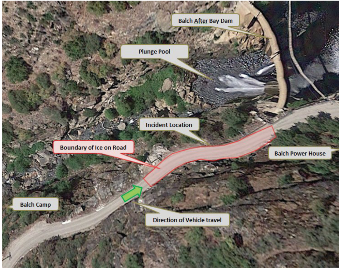
Figure 7 Aerial map showing approximate extent of localized icy road conditions. Vehicle traveled eastward from Balch Camp HQ toward Balch PH. Note: The plunge pool water level was approximately 20 feet higher than depicted in figure 6 & 8 below at the time of the incident due to the spill topping over the Balch A-Bay dam.
