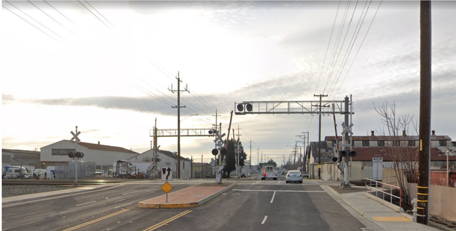
HAZELTON AVENUE CROSSING EAST VIEW
