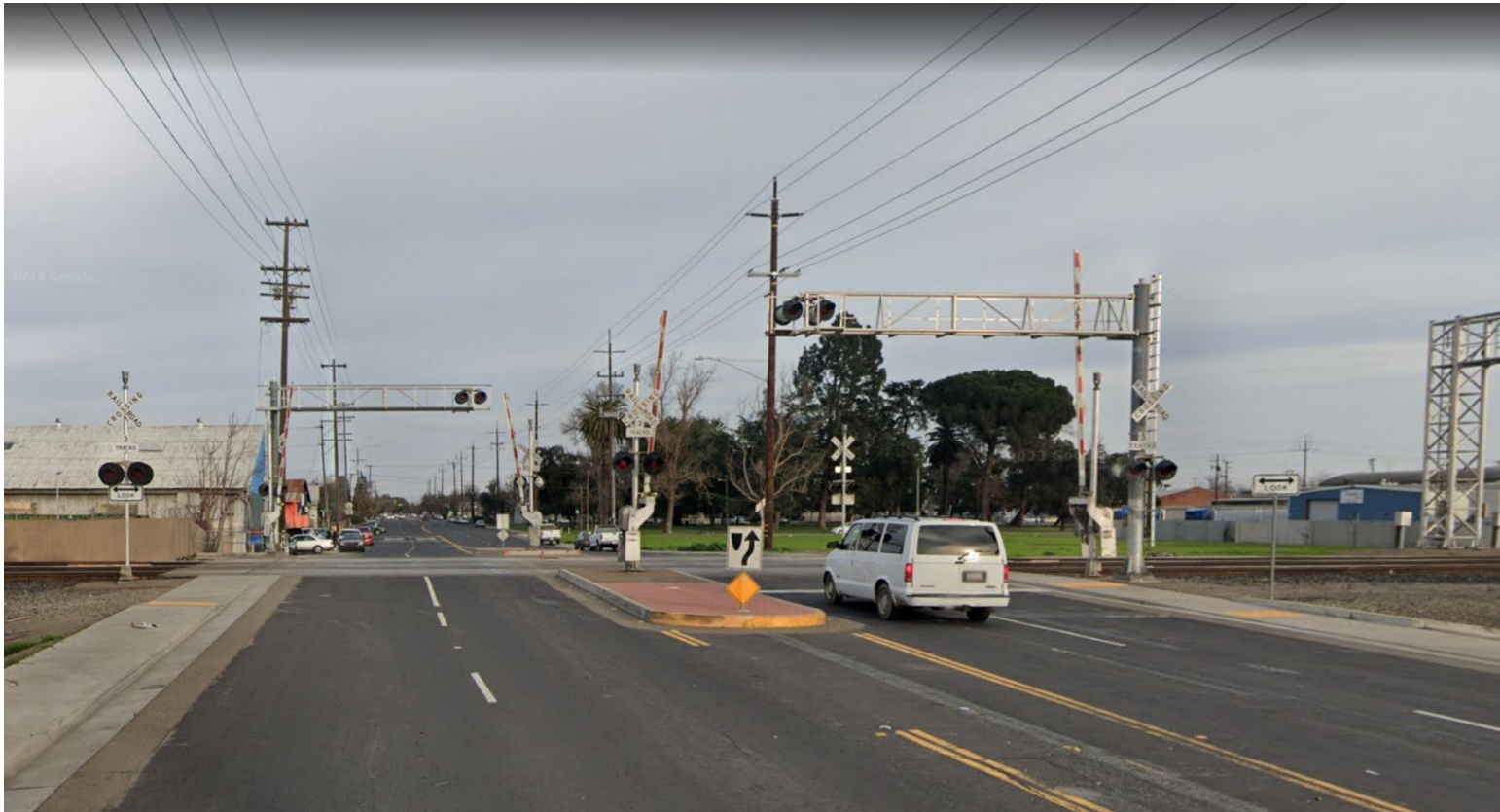
HAZELTON AVENUE CROSSING WEST VIEW
