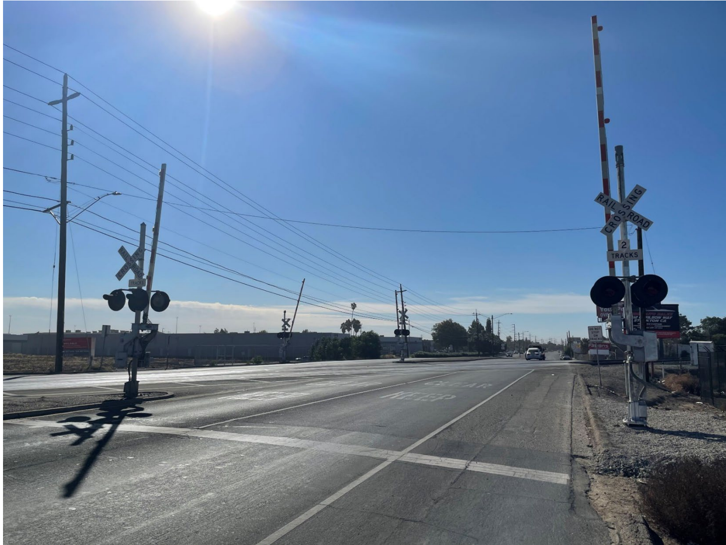
WEST LANE AT-GRADE CROSSING SOUTHBOUND APPROACH
