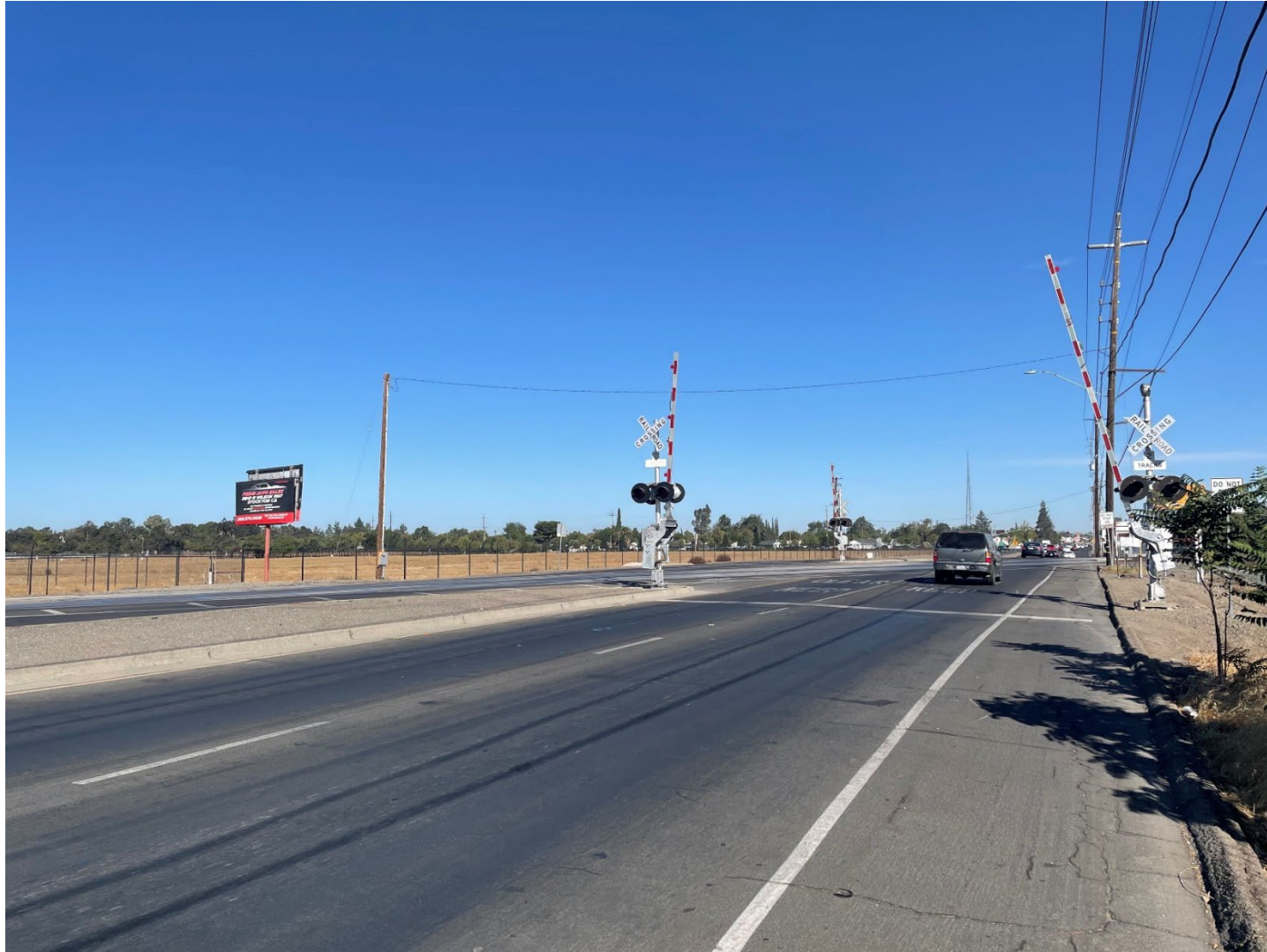
WEST LANE AT-GRADE CROSSING NORTHBOUND APPROACH
