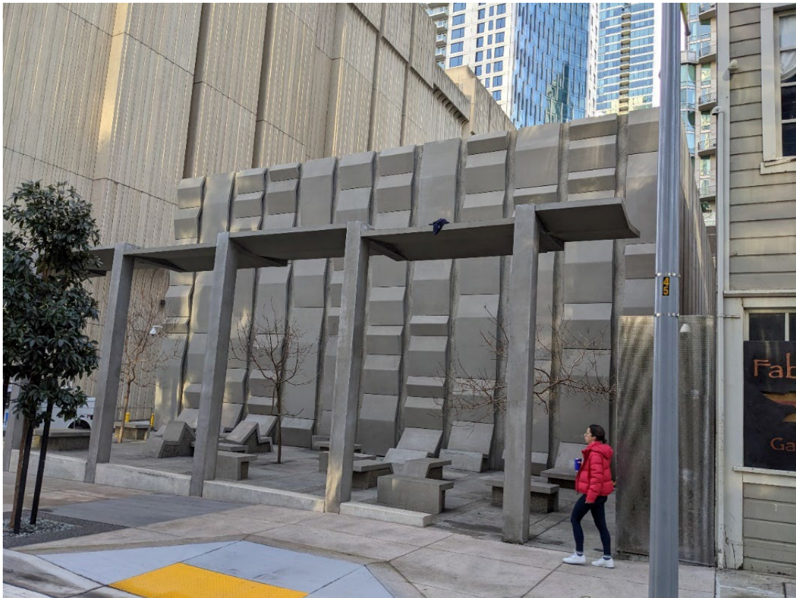
Property 1.2 (Embarcadero Expansion - 425 Folsom St.) View Northeast
