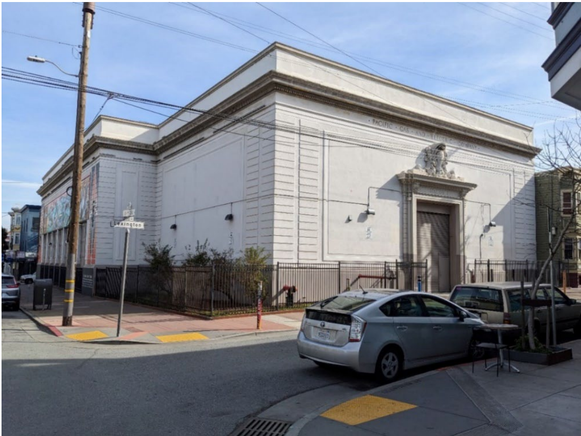
Property 9 (Substation E) View southeast
