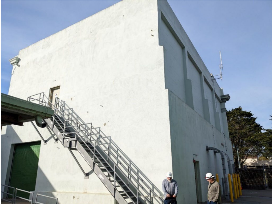
Property 7 (Substation L) Larger Building View Northwest
