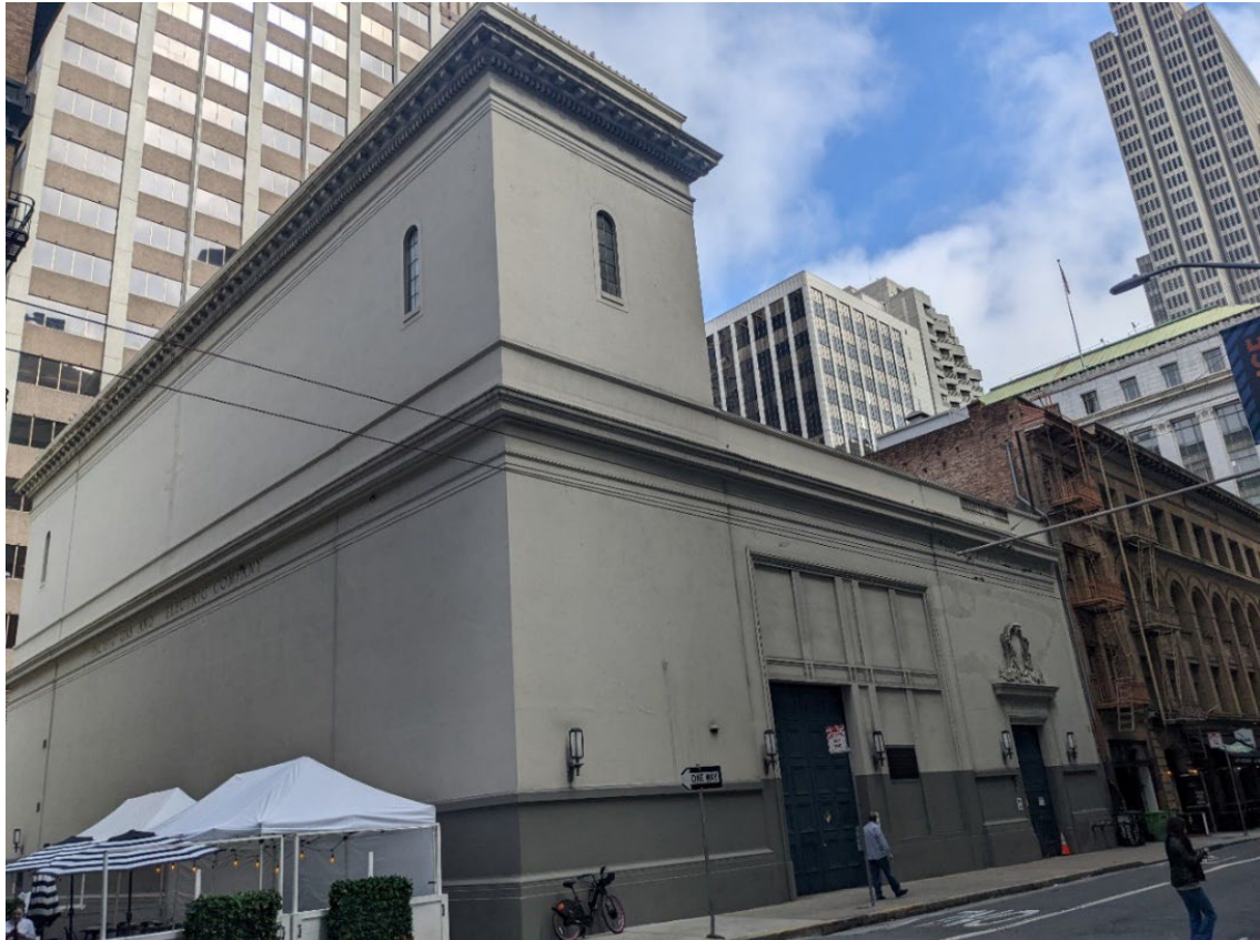
Property 12 (Substation J) View Northeast
