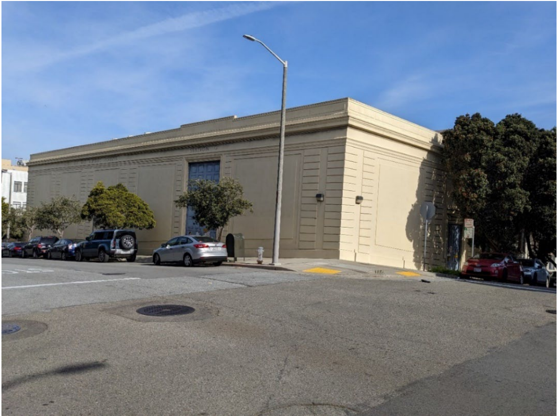
Property 8 (Substation G) View Northeast
