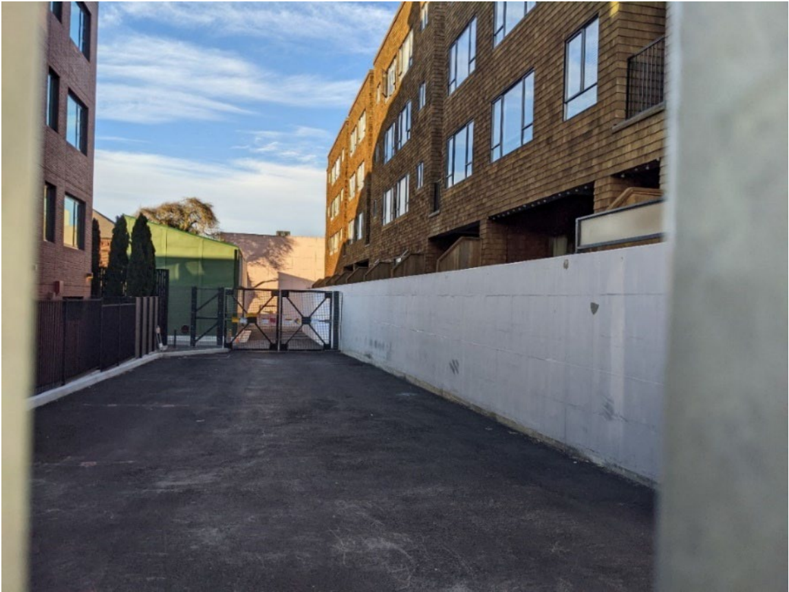
Property 10 (Marina Substation) View North
