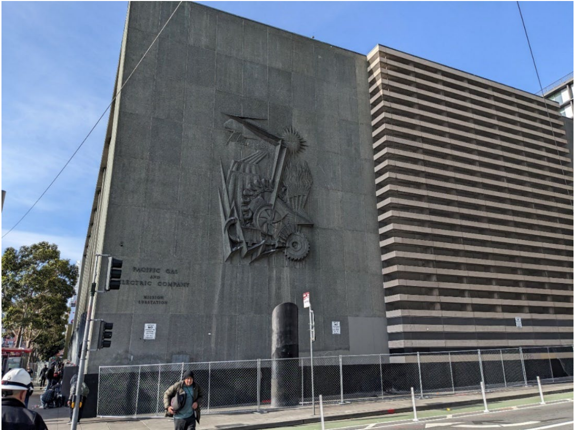
Property 6 (Mission) View West
