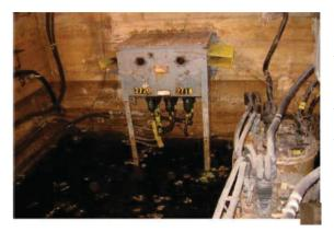
The TGRAM/TGRAL (Transfer Ground Rocker Arm Main/ Transfer Ground Rocker Arm Line) switches represent an extremely antiquated type of underground oil switch. Vendors first introduced these switches in the 1920s. The design was obsolete by the 1960s. PG&E uses its TGRAM/TGRAL switches (1940s vintage) to sectionalize PILC cable. PG&E generally uses a
