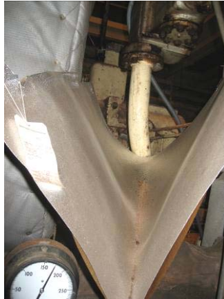
Photo 9. The plant temporarily installed metal sheeting which redirects oil drips away from hot surfaces.
