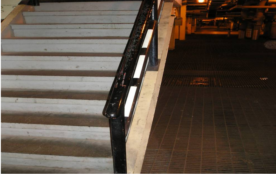
Photo 12. The plant marked this exit stairwell with luminescent tape.
