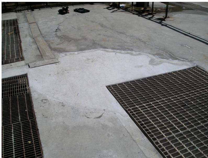
Photo 6. The plant repaired areas of surface delamination.
