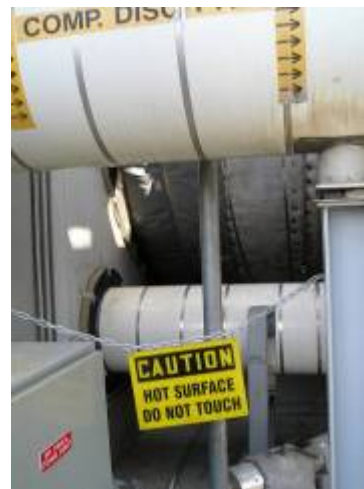
Photo 4: The plant installed new signage and a barrier near the expansion joint vicinity to mitigate burn hazards.
