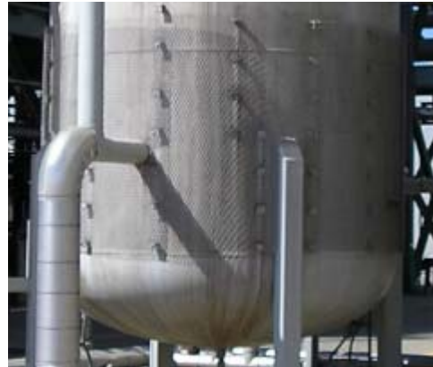
Photo 9: Blowdown tank's lower portion lacks protective barrier.
