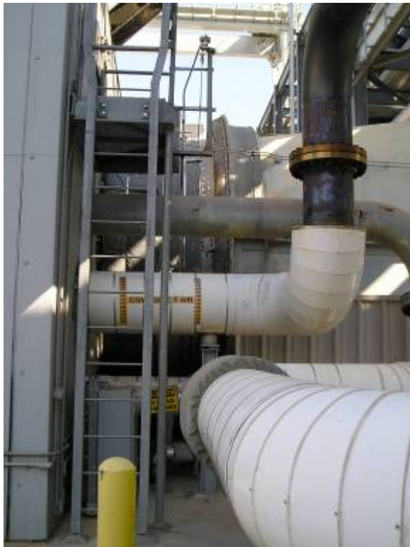
Photo 4: The plant installed new signage and a barrier near the expansion joint vicinity to mitigate burn hazards.
