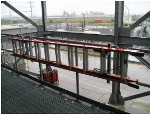
Photo 31: The plant stores ladders on hangers, leaving walkways clear.
