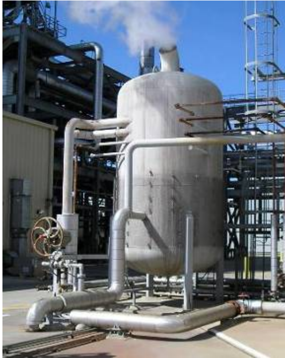
Photo 9: Blowdown tank's lower portion lacks protective barrier.
