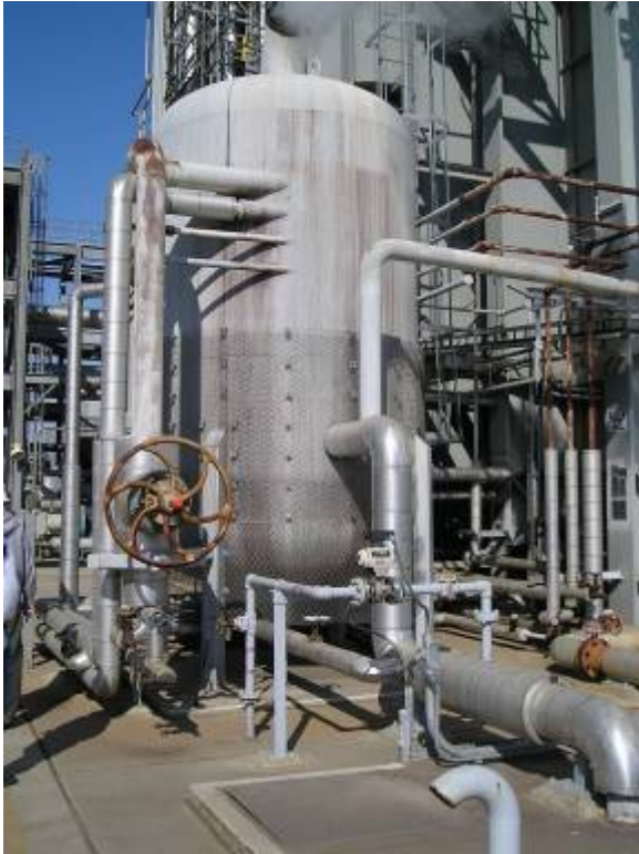
Photo 10: The plant extended the protective barrier to prevent access to the lower portion of the blow-down tanks.
