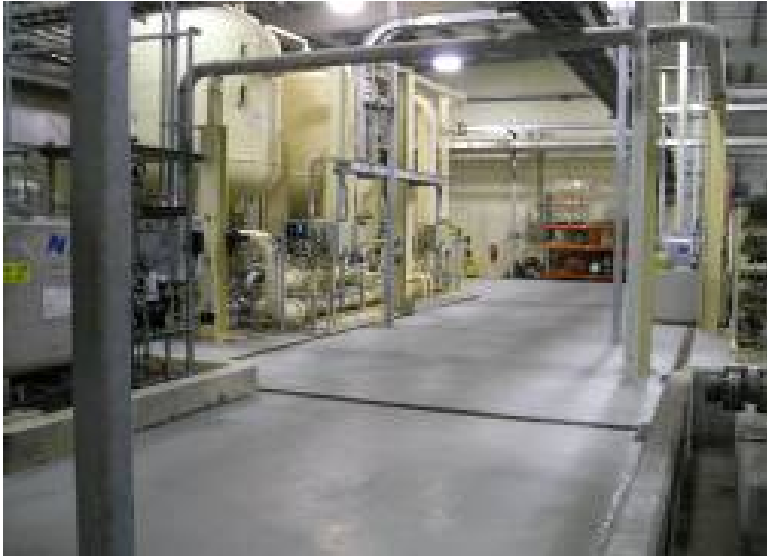
Photo 28: Excellent general housekeeping practices were evident. Here the water treatment area is free of debris.
