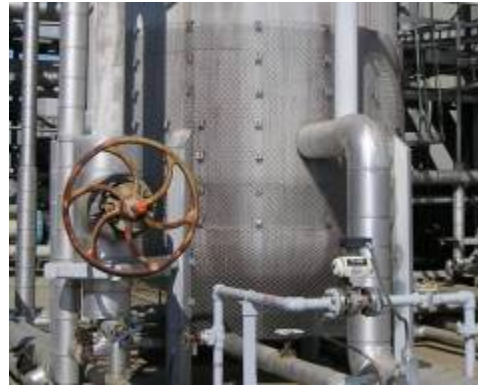
Photo 10: The plant extended the protective barrier to prevent access to the lower portion of the blow-down tanks.
