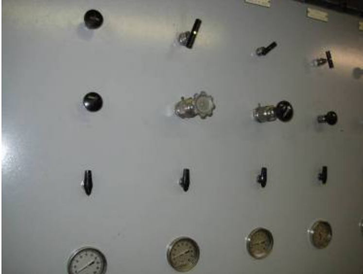
Photo 17: A new valve handle has been installed.
