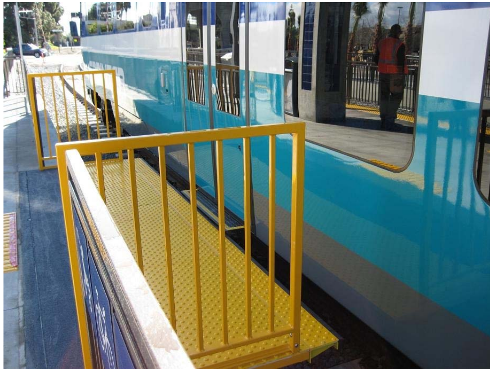
“Wing railings” at High Level Station Platforms With Retractable Gangways
